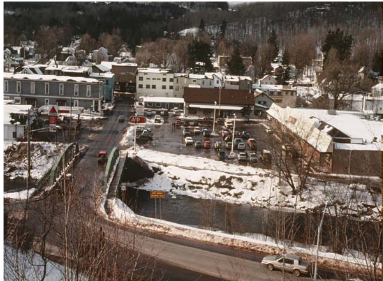
View of Bridge Street entrance Source: M-ARK
